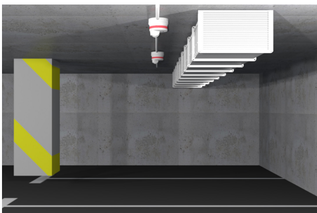
The sensor is obstructed by the obstacle
